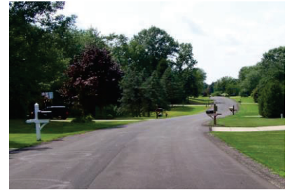
Perry Township Local Road Repaving
