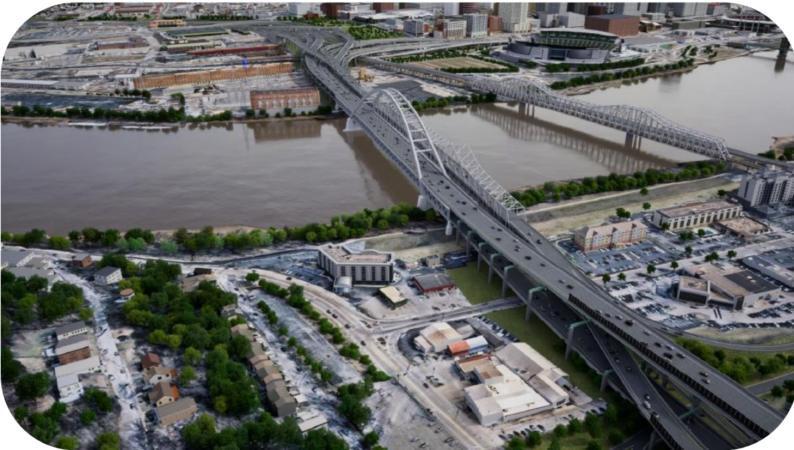
Attribution: Brent Spence Bridge Corridor website. Project view from Kentucky looking north.
